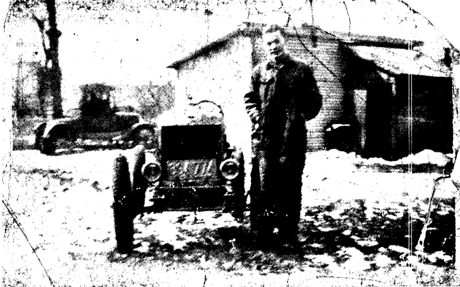
Mount Pleasant Man Builds a Fast One "Small but speedy is the way Frank Janesko describes the car which he built during his spare time. Only 36 inches wide with a 69½ inch wheel base, it can travel at a rate of 75 to 80 miles per hour." Pittsburgh Gazette, 1925.
